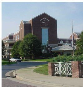
Presbyterian Hospital Matthews
